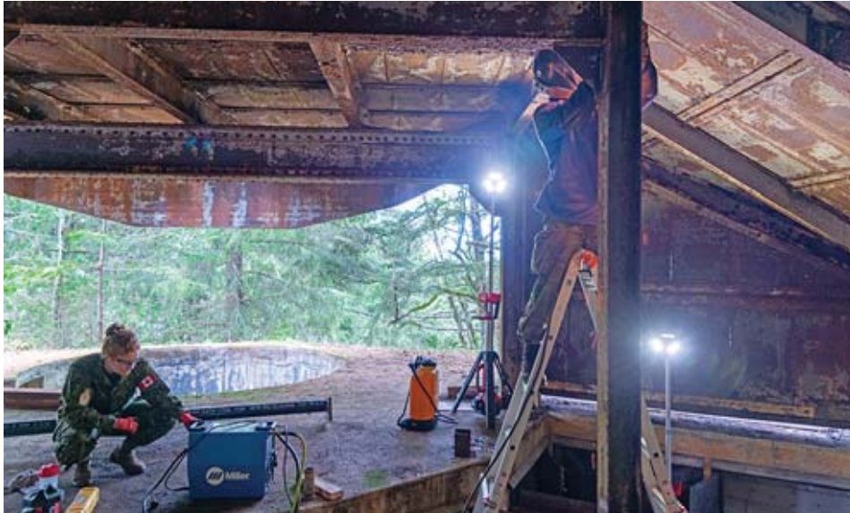
Master Corporal David Low, 192 Construction and Engineering Flight, Aldergrove, removes bolts from a support beam in the Yorke Island Fortress.
