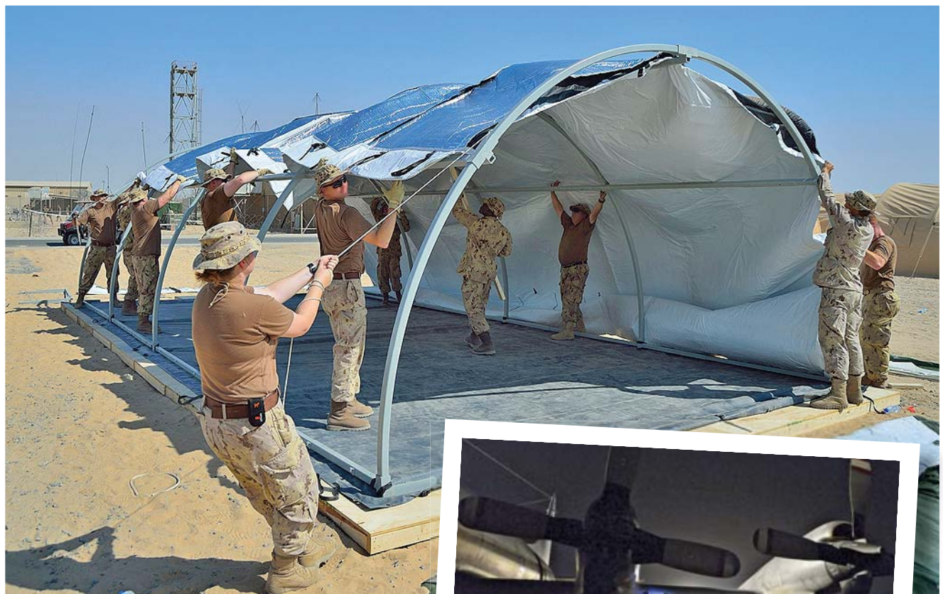
Before covering a shelter with a weather protective sheet October 19, Canadian Armed Forces members drape a thermal layer over the framing of a climate controlled shelter that will be used by the Canadian Air Task Force in Kuwait. Canadian Forces Combat Camera
