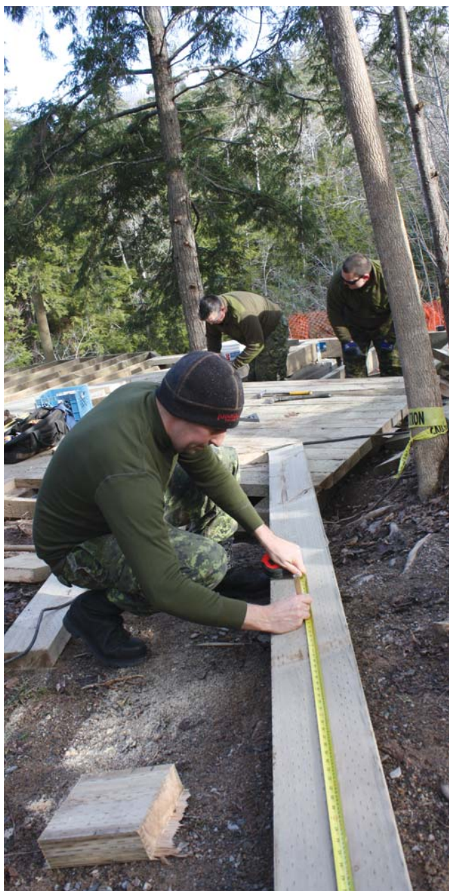
Corporal Tim MacDonald prepped the boards for placement in the deck, as crews worked December 11.
