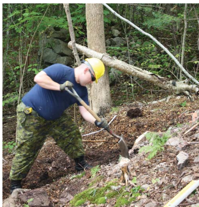
Corporal Ian Delafontaine at work digging footing holes in rough terrain: hole number four of the day – of 18 on the plan....
