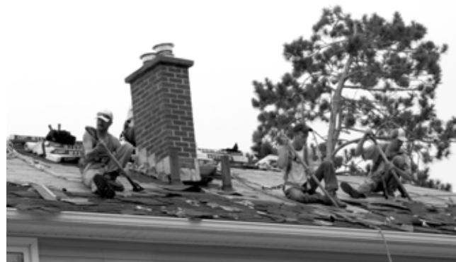
A roofing crew bright and early, reshingling in the RHU neighbourhood.
