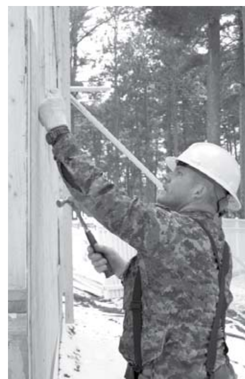
Corporal Mike Probert, nailing exterior sheathing in place, is the site foreman for Construction Engineering Flight's current project, a replacement garage at the wing commander's residence. S. Keddy
