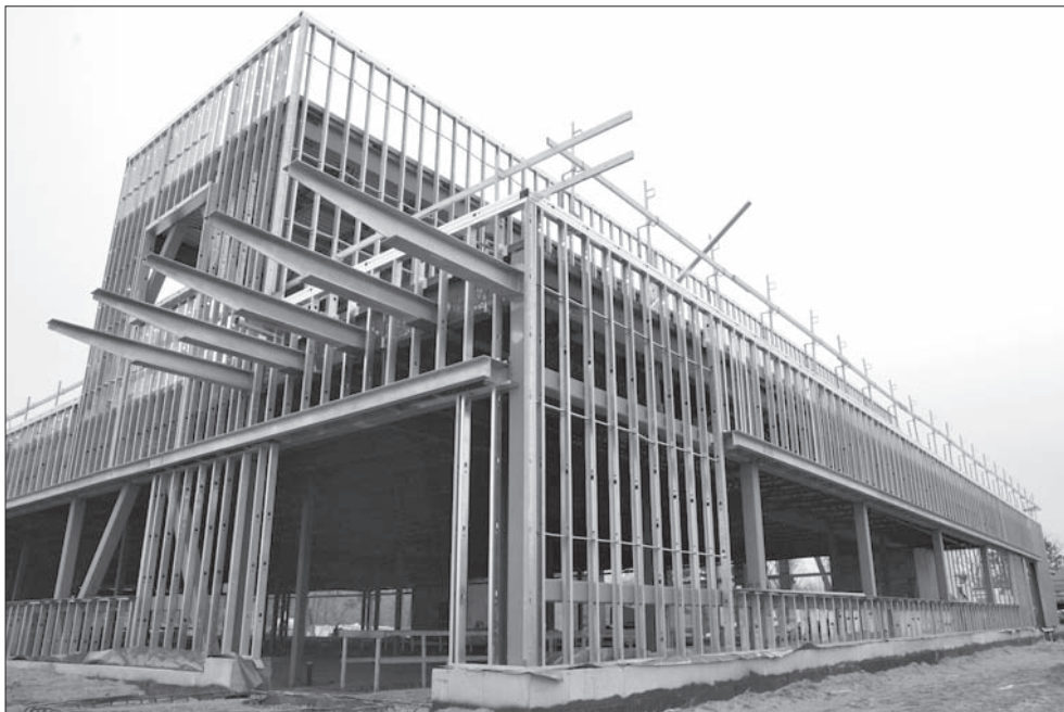
Exterior views of the Health Services building during construction showing steel super structure.
