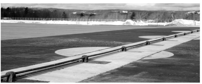
The new barrier arrester cable, extending over the 14 Wing runway.
